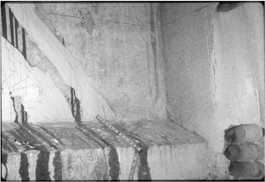
Figure 5. Some preliminary repair implemented by injecting polyurethane foam in the cracks is seen to be ineffective at I-565 highway bridge girder in Huntsville.
