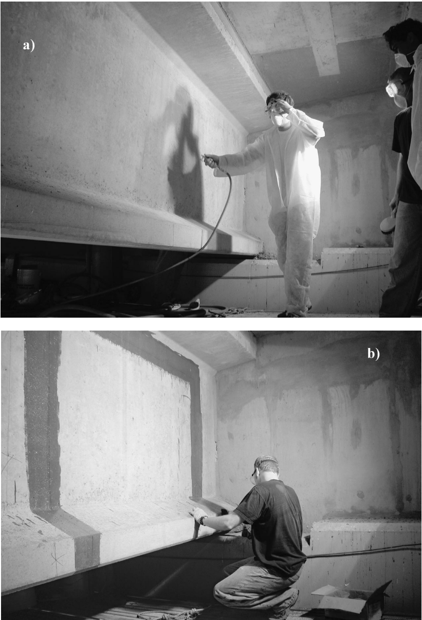
Figure 16. (a) Surface preparation and (b) pre-priming of vacuum bag sealant tape zone.
