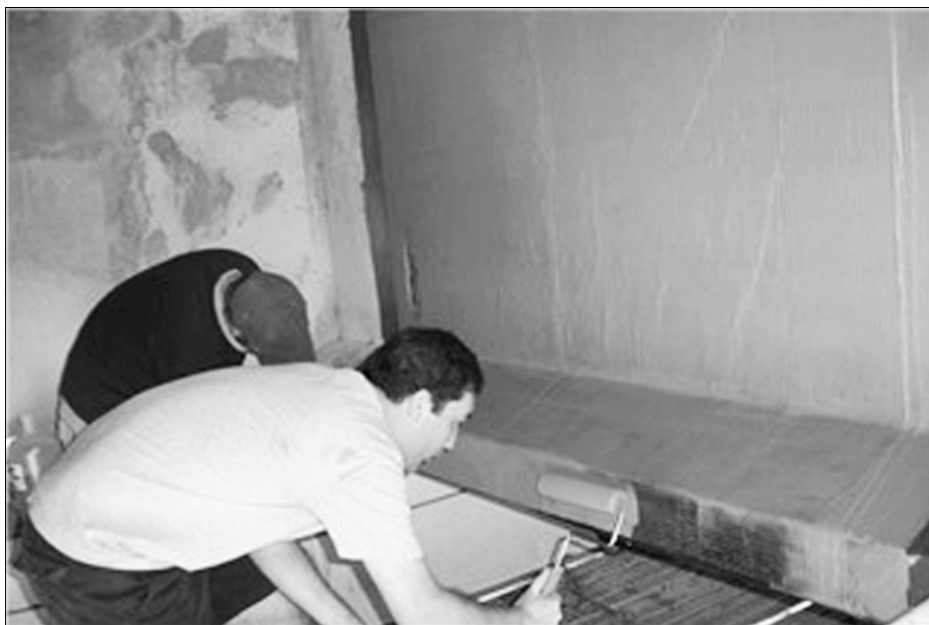
Figure 22. Latex based coating application.
